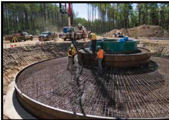
Figure 2. Example of a foundation. Image courtesy of Don Pettit, Peace photoGraphics.
