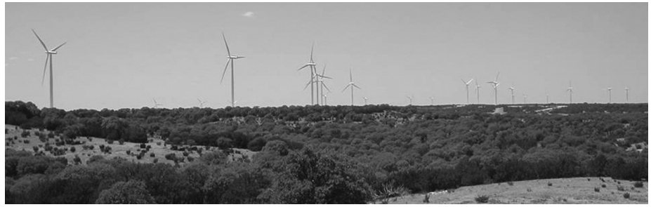
Horse Hollow Wind Energy Center, 20 miles southwest of Abilene in Taylor County and Nolan County, Texas. Photo courtesy of Epsilon Associates Inc.
